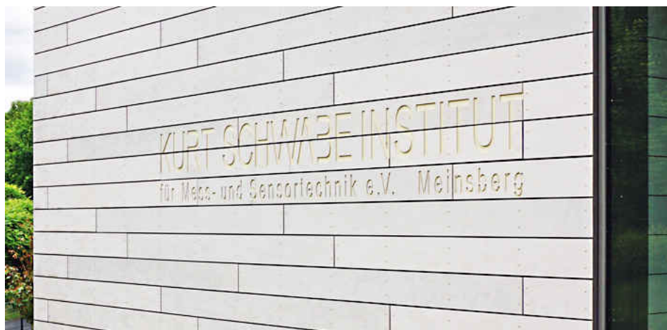
Building detail of the Kurt Schwabe Institute for Measurement and Sensor Technology Meinsberg (KSI Meinsberg)
